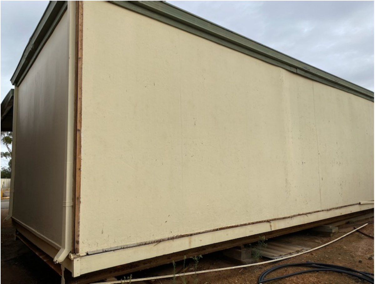
Deport office side 9.3m x 4.2m
