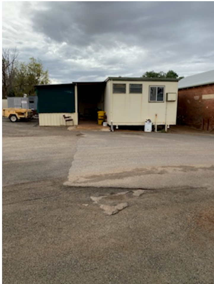
Depot office front 4.2m
