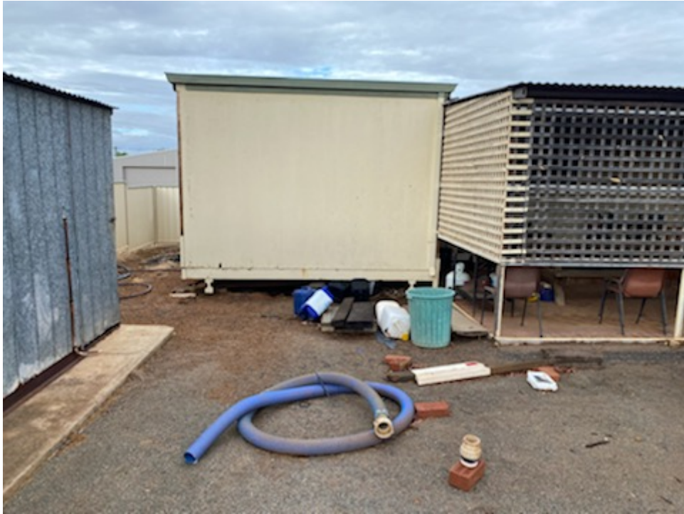
Depot office rear 3.6m x 8m
